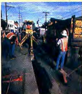
CARVING A TRENCH DOWN THE MIDDLE OF A LOS ANGELES-AREA STREET TO MAKE ROOM FOR MFS'S FIBER LINES.
